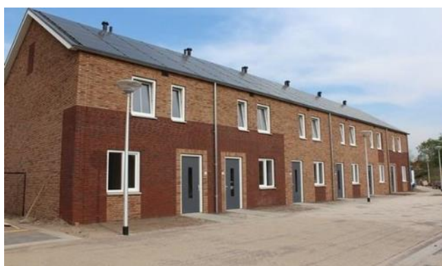
Figure 5 New dwellings with solar panels that are gas free from Woningstichting Woningbelang 10
